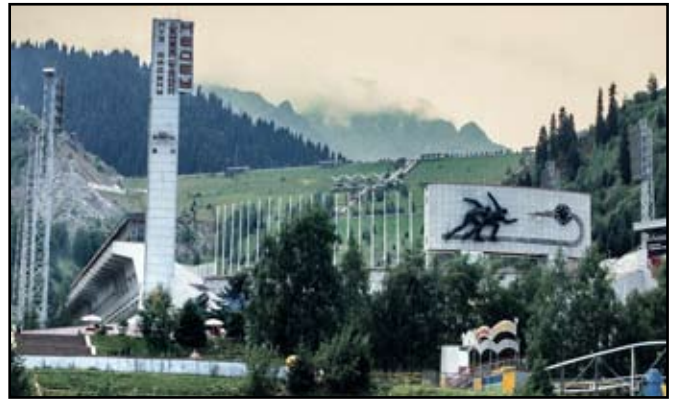
The Medeu ice stadium protected below the downstream face of the rockfill dam which acts simply as a catch for debris flows.
