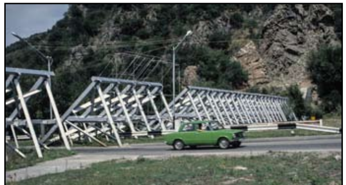
Upstream face of one of the more modest debris-catch-barriers downstream of the Medeu dam.
