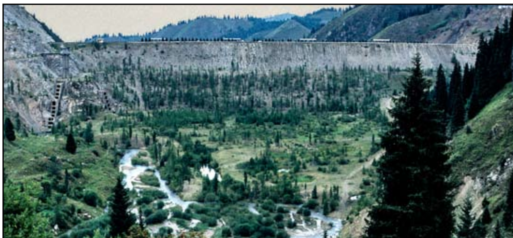
Upstream face of one of the more modest debris-catch-barriers downstream of the Medeu dam.
